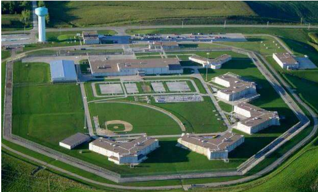
NEWTON CORRECTIONAL FACILITY MEDIUM SITE
