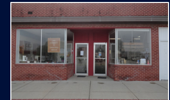
Creston Office 119 N Elm St Creston, IA 50801 (641) 782-8556
